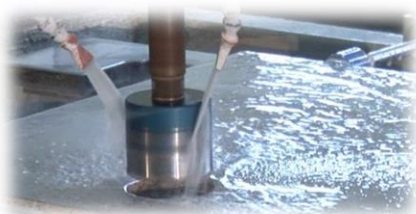
Wet drilling with core bit
